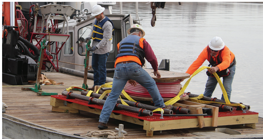
COST-EFFECTIVE DOCK AND JETTY ICCP SLED Sturdy timber frame makes transporting and placing units easier than steel sleds.
