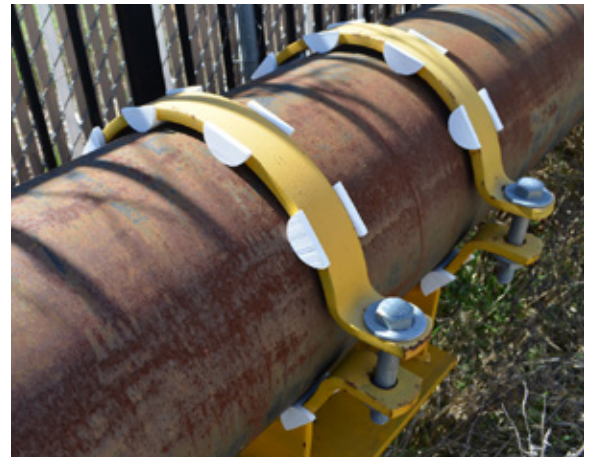
FOR GRINNELL CLAMPS Clips can be held in place with double-sided tape during installation.
