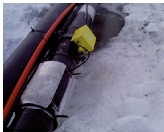
ALASKA MA-1 monitor installed on a bracelet anode in Alaska.
