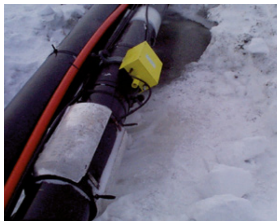
ALASKA MA-1 monitor installed on a bracelet anode in Alaska.
