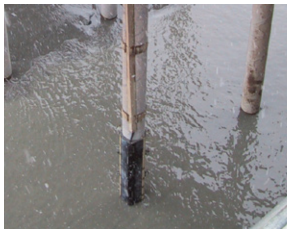
Raparound in situ After two brutal Alaska winter freezes, performance is unaffected.
