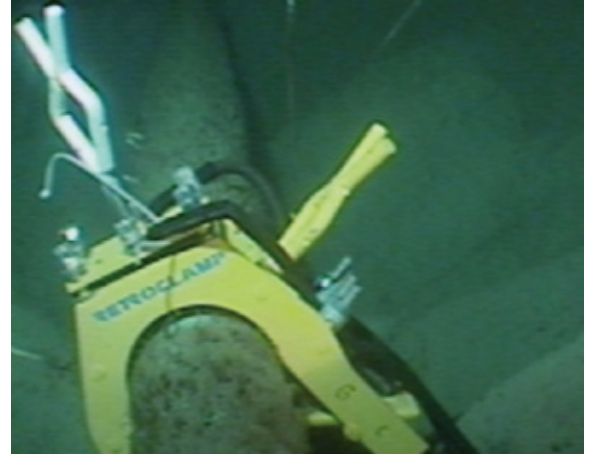
ROV INSTALLATION RetroClamp on a deep-water flowline, retrofitted by ROV.
