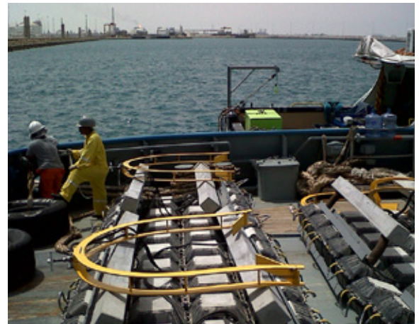
A SPECIAL DESIGN FOR QATAR Aluminum anodes on this job were cast on the outside of the RetroMats.
