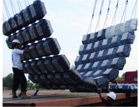
ANODES ARE CAST INTO THE CONCRETE SEGMENTS The wire rope core of the mat provides a low resistance anode array.
