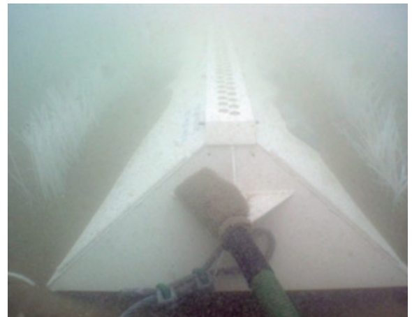
INSTALLATION VSE anode installed on bottom: it is already beginning to silt over
