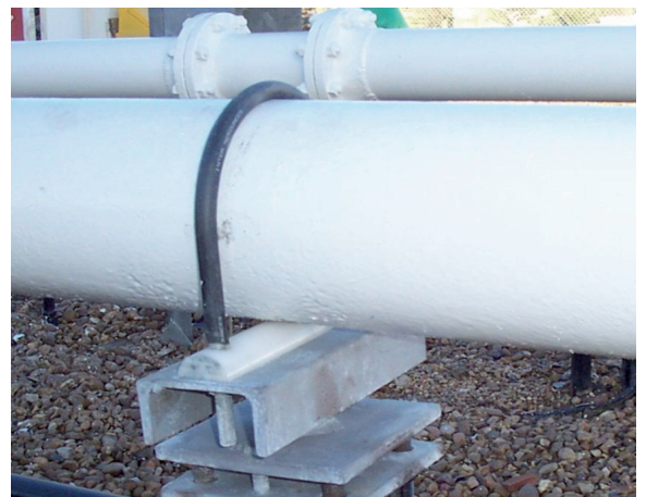
Offshore Nu-Bolts on pipe run at (+) 10'0" elevation on an offshore platform.
