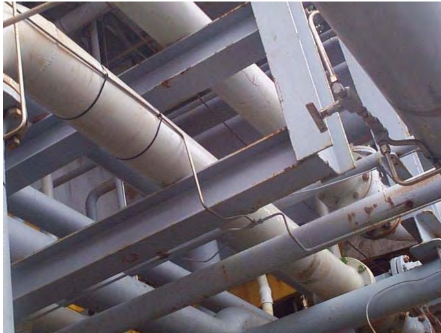
Figure 1. Typical I-Beam Pipe Support
