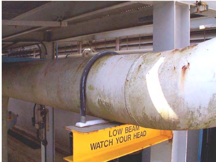
Figure 13. Typical Rod – U-Bolt Stand Alone Support
