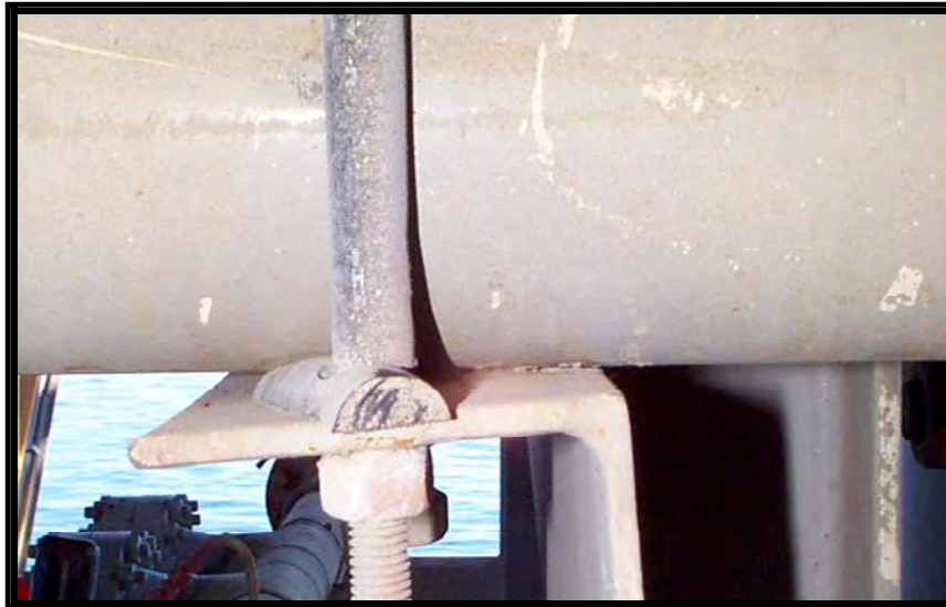
Figure 17. Low Grade Material Copies Crush Under Load
