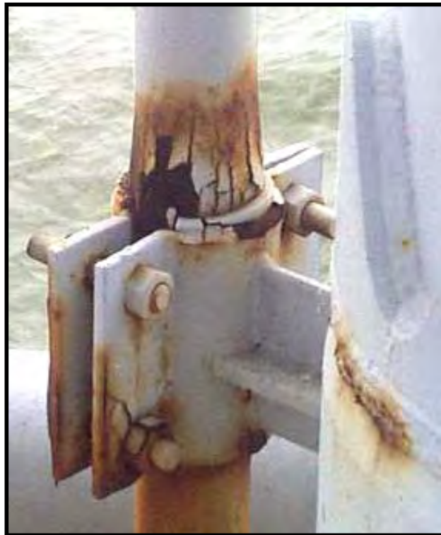
Figure 4. Full Saddle Clamp
