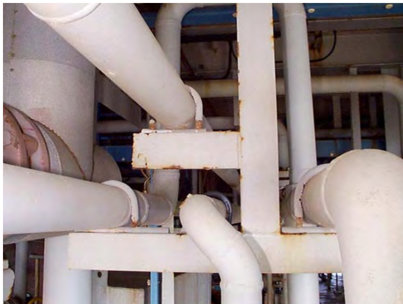
Figure 16. More Rod Bolt Combinations 13 Years Offshore
