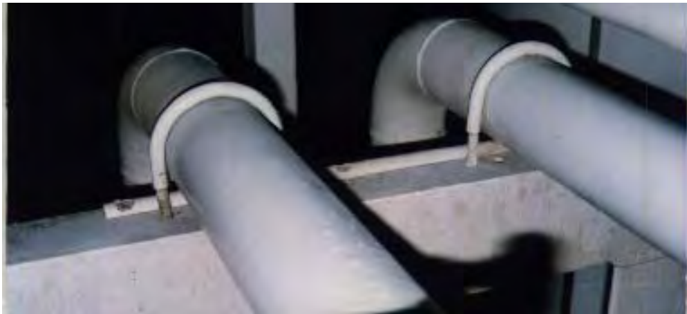
Figure 12. Rod Installed as Beam Dressing
