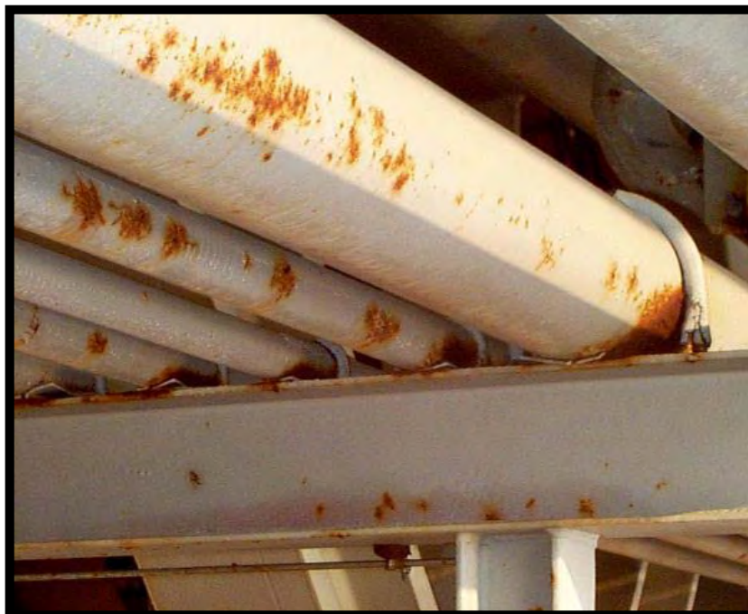
Figure 2. U-Bolt Stabilized Beam Supports
