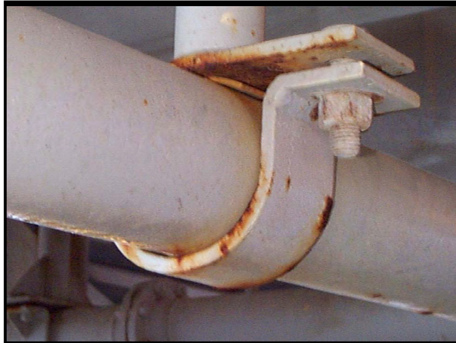
Figure 3. Typical Half Saddle Clamp
