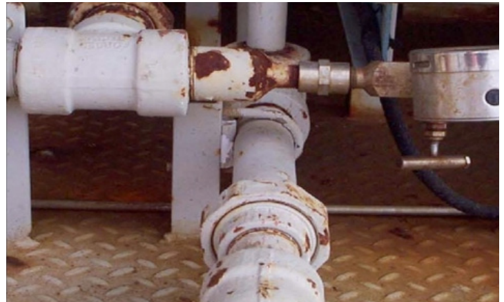
SMALL PIPES, BIG HEADACHE I-Rod is particularly effective on small-diameter screwed piping, which has the highest maintenance cost per square foot on the platform. This smaller piping is shown in the three adjoining photos.
