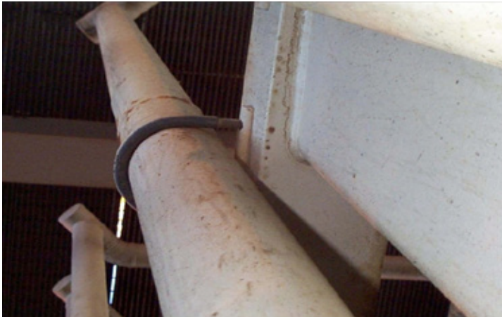
KEEPING IT FLOWING A typical Nu-Bolt on a vertical section of a flowline.
