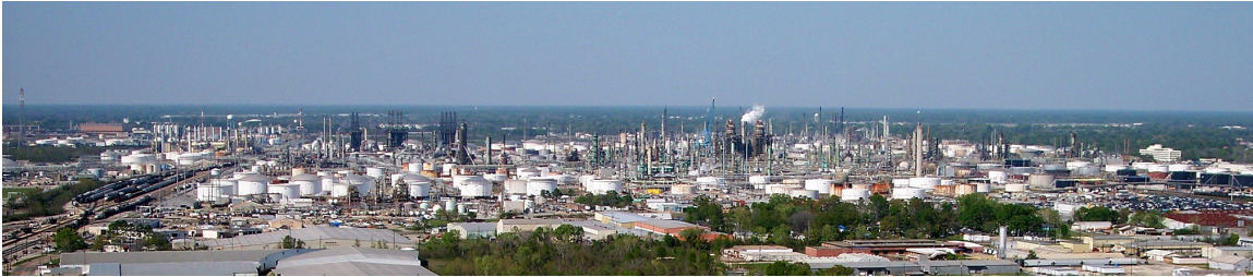
ExxonMobil refinery in Baton Rouge. Photo by Adbar
