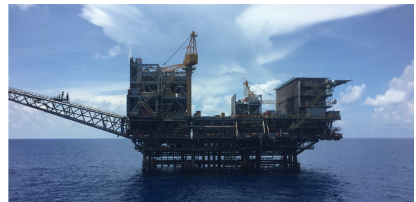
PLATFORM FOR RETROSLED REMOTE ANODE RETROFIT
