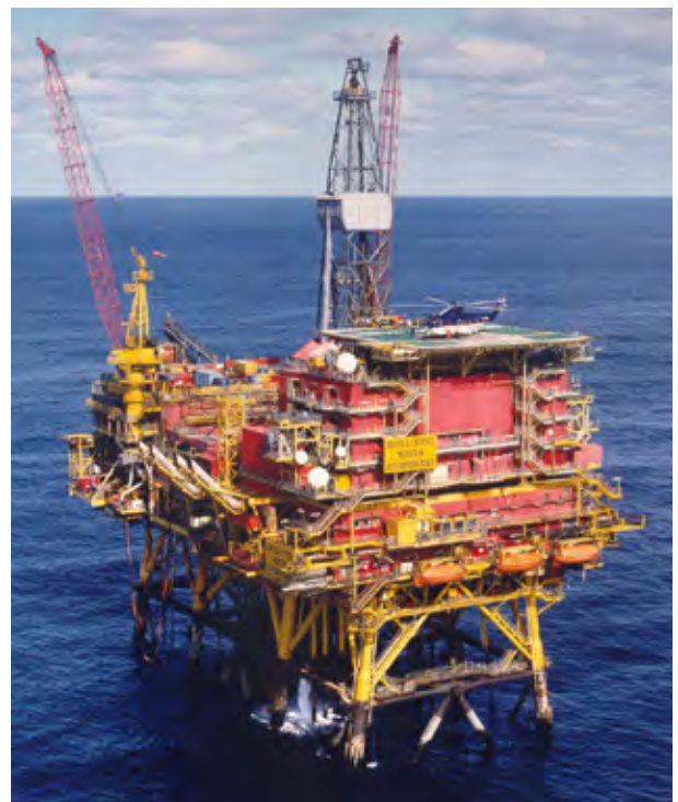
FIG. 1: A 20-YEAR LIFE EXTENSION WAS NEEDED The North Sea platform is in 160 meters of seawater
