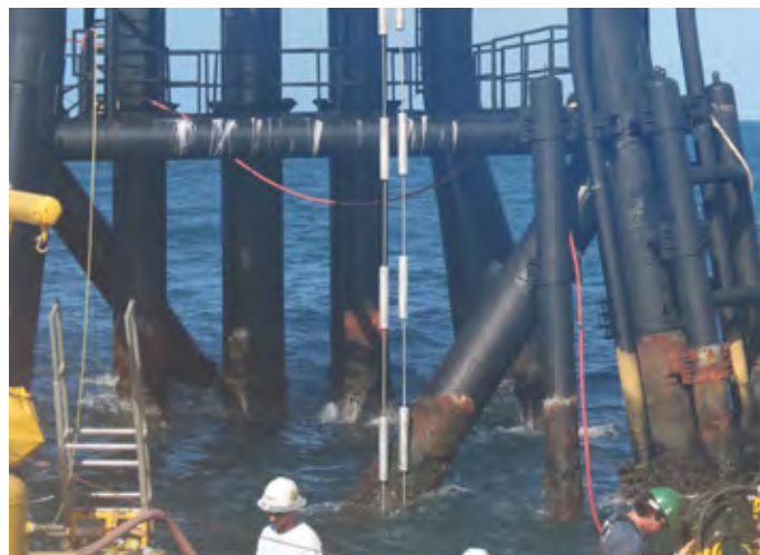
FIG. 15: SKIRT LINK INSTALLATION The retrofit and inspections took four days offshore
