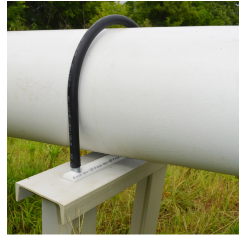
I-Rod® eliminates the crevice by minimising the contact area and allowing any moisture to evaporate. It's also much easier to inspect.
