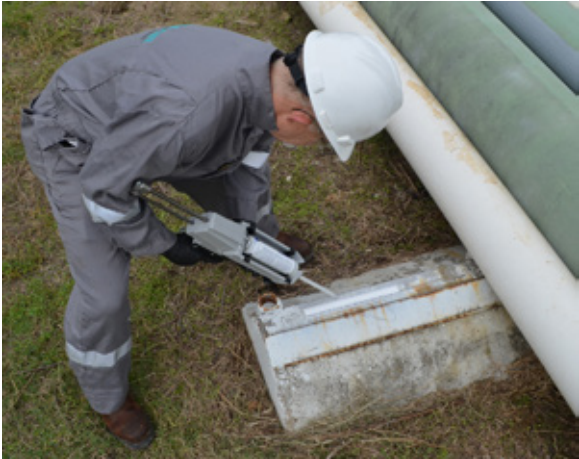
FORMING A BOND I-Rod Adhesive will permanently hold I-Rod in place when bolting is not an option.
