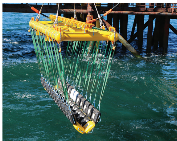
A BOATLOAD OF MATTRESSES WERE NEEDED Luckily, placing them took just 20 minutes each.
