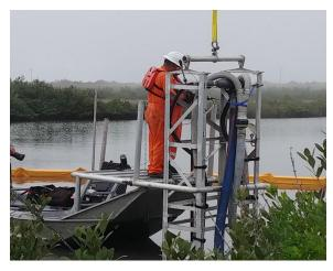
TAKING AIM The PET™ lowers onto the pipeline as it clears away the mud cover.
