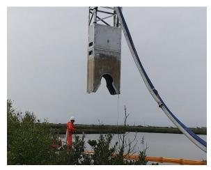
GETTING POSITIONED The PET™ is lowered into the guide frame using a crane
