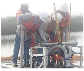
FULLY EXCAVATED The PET™ rests on the pipeline just before the RetroClamp™ is installed.
