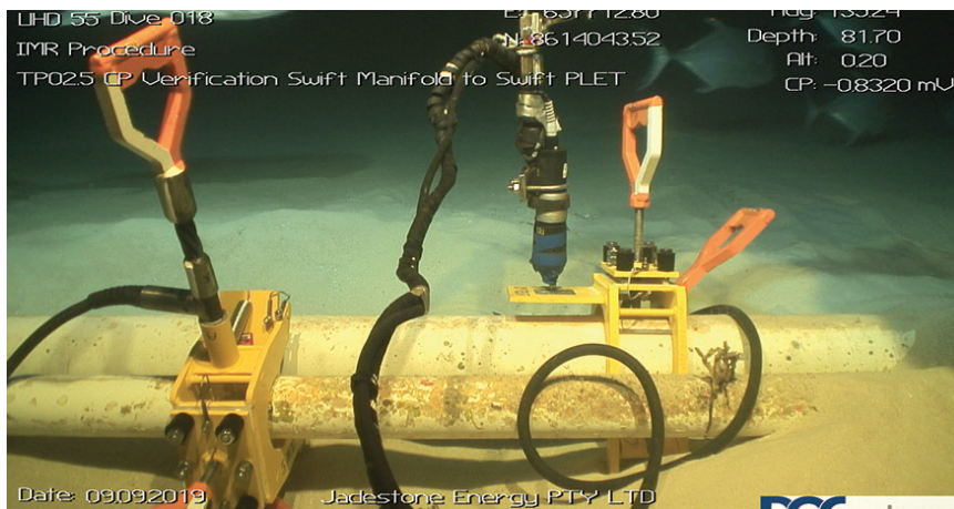
FLOW LINE BONDING A tieback cable from a 4" RetroClamp™ to the test station bonds the gas lift piggyback to the host flow line.
