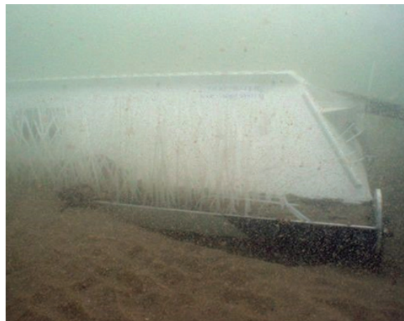
THE VSE ANODE INSTALLED
