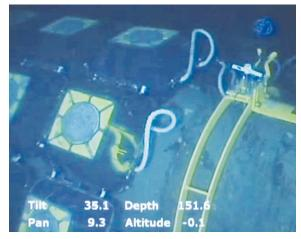
MAKING THE CONNECTION The mats are electrically connected to the pipeline using RetroClamps<sup>TM</sup>.
