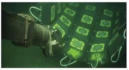
PRECISELY POSITIONED ROVs assist in positioning the mats when they're lowered into place.
