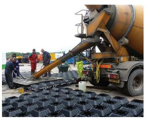
ADDING SOME WEIGHT Local crews fill the RetroMat<sup>™</sup> shells with concrete before deployment.
