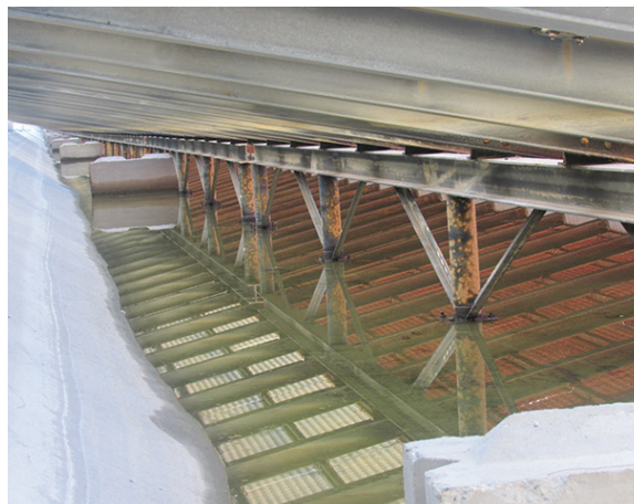
CORROSION CHECK-UP Technicians took pitting measurements and checked for electrical continuity.
