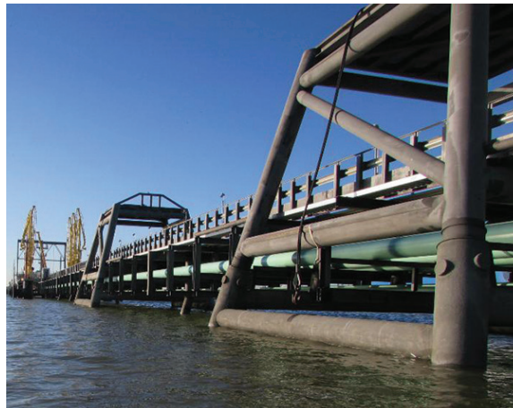
KEEPING CORROSION AT BAY IN GALVESTON BAY A hybrid system was determined best for the dock facility..
