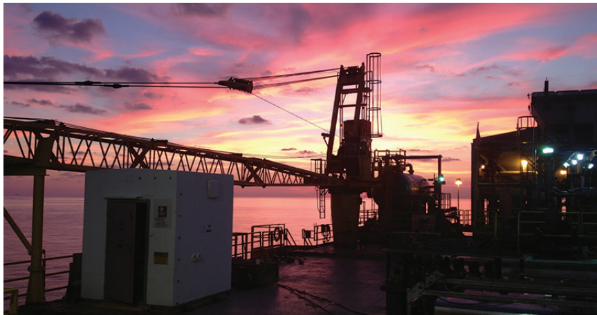
NEW LEASE ON LIFE The dual RetroBuoy™ will provide a 20-year life extension for the Ewing Bank 305-A platform.
