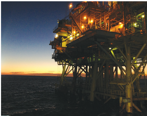
AN EIGHT-LEG FIXED STEEL JACKET The platform sits in 300 ft of water in the Gulf of Mexico.
