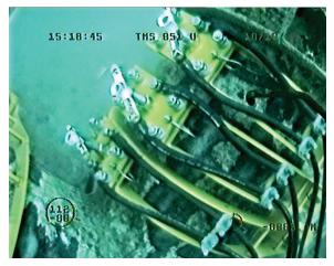
**AMPS THROUGH THE CLAMPS** RetroClamps $^{TM}$  electrically attach the RetroPods $^{TM}$  to the structures.
