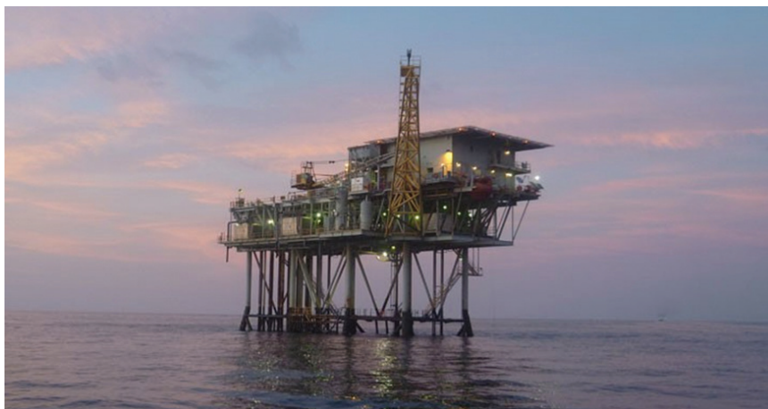
EI-295-AD The platform sits in 220 feet of water in the Gulf of Mexico near the Louisiana coast.
