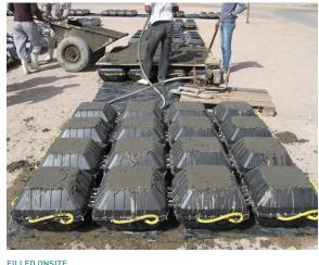
FILLED UNSITE Ballast mattresses are filled with concrete onsite to save on shipping expenses
