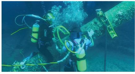
14 RETROPODS™ IN 20 HOURS Divers placed the clamps and confirmed CP levels once the new anode sleds were attached.
