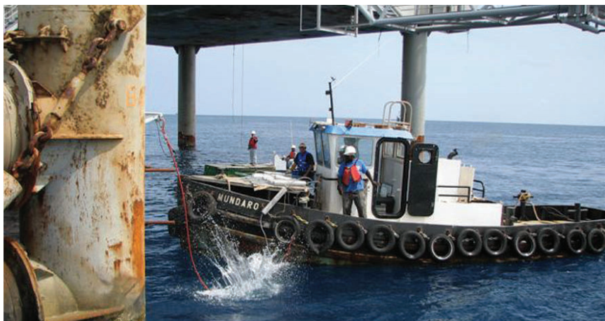
EASY ACCESS Links were installed from a work boat without using divers..
