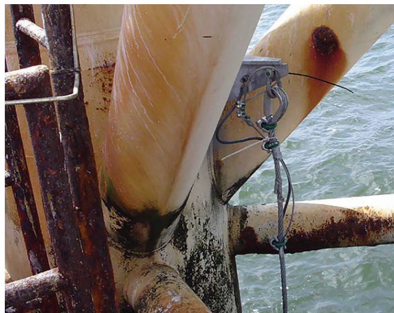
RETROLINK™ IN PLACE RetroLink™ anode strings are guaranteed to survive hurricanes.
