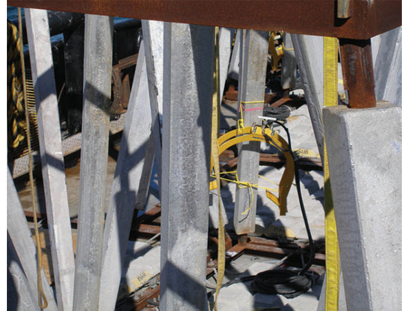
THE POD SQUAD Five structures required deployment of 94 RetroPods™.
