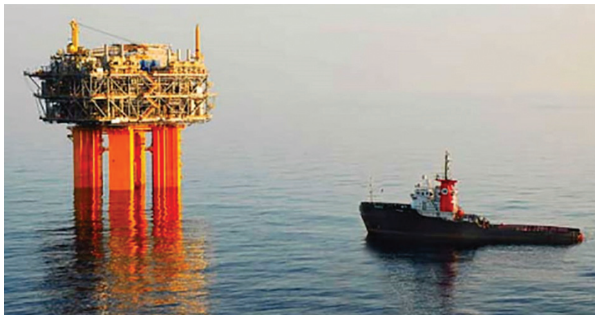
ROUGH NEIGHBORHOOD The platforms sit in 4,400 ft of water in the Gulf of Mexico in an area with high sub-surface currents.
