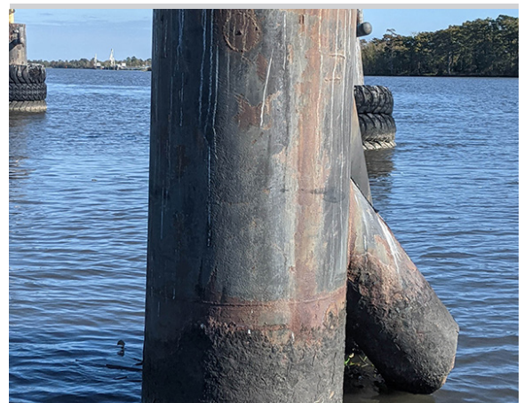
PILING ON MORE CP
