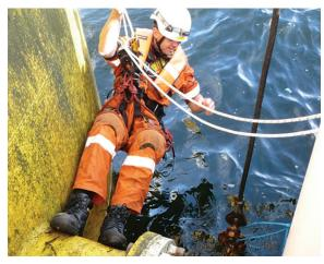
NEEDED A BOOST Four RetroLink™ anode strings were added to beef up inadequate CP levels.
