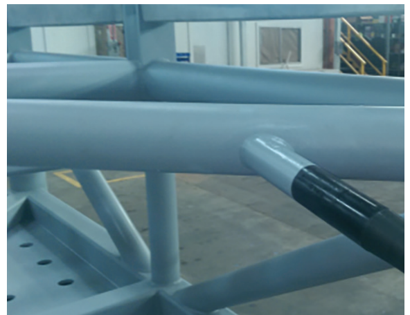
TUBULAR DESIGN High-strength piping was used in the construction of both sleds.
