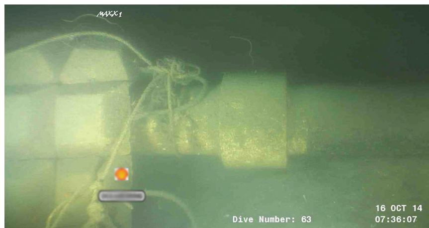
THE INSULATOR FLANGE Crude can pass through, but not cathodic protection. Deepwater's jumper system fixed that problem.
