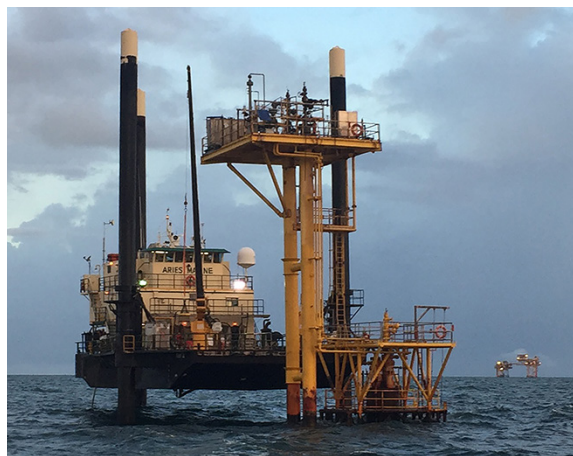
THE WORK BOAT The installation was completed using this jack-up boat.
