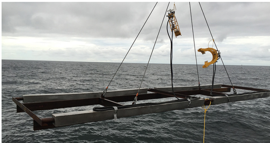
SLEDS HEAD FOR SEABED Four RetroSleds™ will provide cathodic protection for the two pipelines.
