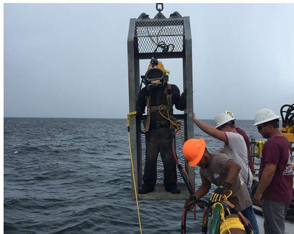
DIVERS DOWN The RetroClamps™ were placed onto the pipelines by divers.
