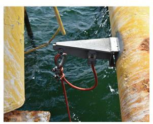
ATTACHMENT IS VIA HANGOFF WELDED TO STRUCTURE At least two of the anodes lie in the mud after installation.
