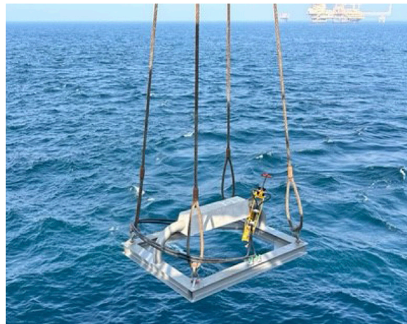
AN ANODE SLED BEING LOWERED INTO PLACE The RetroClamp™ will electrically tie it to the pipeline.
