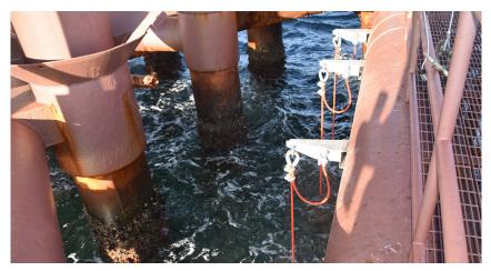
RAPID INSTALLATION The RetrLinks™ were hung from horizontal stand-offs welded to the structure.
