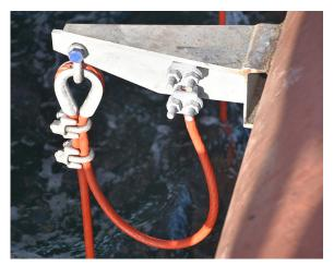
ATTACHES ELECTRICALLY AND MECHANICALLY ABOVE THE WATER LINE They're usually installed from a small vessel without using divers.
