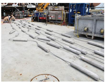
RAPID INSTALLATION All 14 anode strings were installed in only 9 hours.
