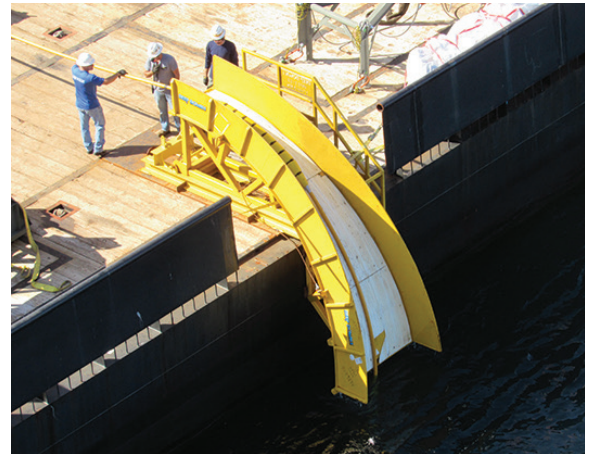
A MODEL INSTALLATION Optimal RetroBuoy placements were determined by CP modeling beforehand.
