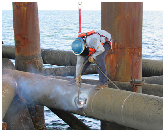
RUGGED ATTACHMENT Hang-offs for the RetroLinks™ were welded onto the structure.
