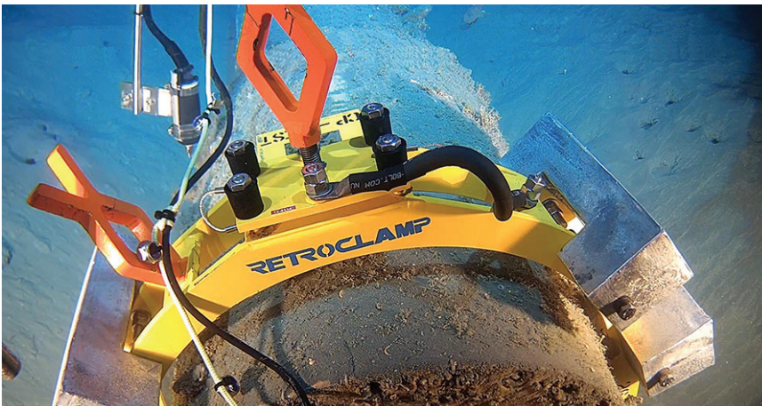
RAPID INSTALLATION A RetroClamp™ is an efficient, reliable method of replacing spent anodes on underwater pipelines and structures.
