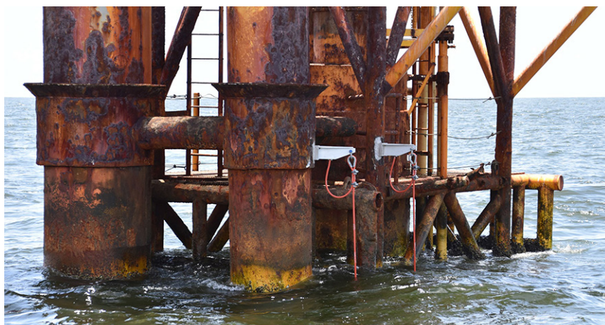
THREE RETROLINKS™ PROTECT THIS STRUCTURE IN 44' OF WATER Sixteen structures were retrofit in eight days.
